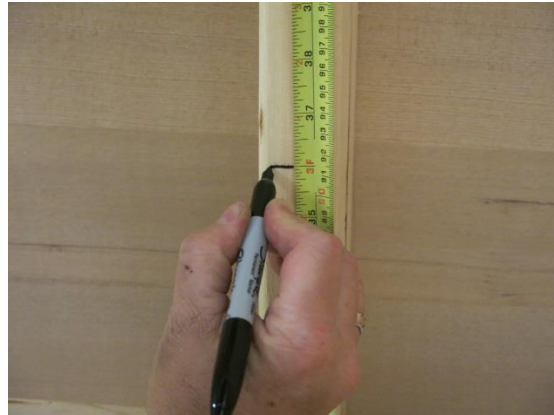
Photo 03. Marking the height of the IS panels.
