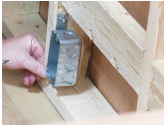
Photo 04. Mount just above bottom framing plate so all boxes will be below the lower bench. Make sure the box is positioned to be flush with your finished wall surface.
