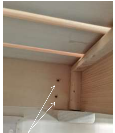
Two screws under the return bench
