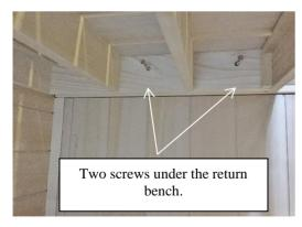
40. Install the screws with washers under the bench upper return through the frame to the main upper bench.
