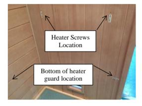
28. Assemble and install the wood heater guard around the sauna heater using the 1 1/8" screws provided. The heater guard location is marked on both walls with a label. Place the bottom of the heater guard to cover the label on the walls and secure into location.
