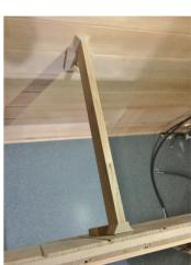
33. Install the bench brace from the back of the Bench Skirt to the back wall.
