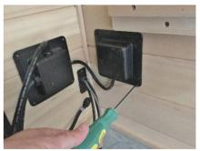
9. Place CB Box on the floor for easy access. Remove the cover to access the electrical connections.
