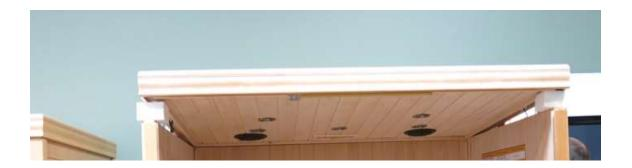
• Once the Ceiling panel is lined up directly above the Wall panels; insert the wires harnesses from the wall panels into the holes in the Ceiling panel.
