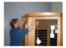
• Once the Ceiling panel is lined up directly above the Wall panels; insert the wires harnesses from the wall panels into the holes in the Ceiling panel.
