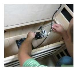
• Locate the electrical switch on the black Master Control Box and ensure the switch is on.
