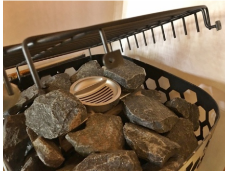
BWT tank, tank lid, and the vent cover installed and the rocks placed around the tank.
