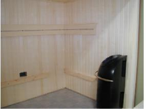
First secure the bench supports to the walls. There will be a pencil mark and labels showing where the top of the supports will be placed. Note: the heater should be hooked up before beginning the bench installation. Once all supports are in place, install the decking (bottom bench) starting with the heater side. The hole for the bowl/dish may or may not be in the bench depending on the room configuration. Next install the other side decking.
