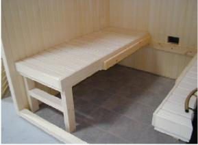
Third, put the middle decking into place. Once the decking is set, the upper (modular) benching can be placed on top. (Middle deck is removable for cleaning.)
