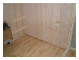
Step 1: Prior to installing the all-glass front, start on the right side of the room and note that the bench supports on the back wall have been pre-installed.
