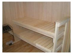
Step 6: Place the top bench on the supports as you did with the bottom bench and secure in a similar manner as the bottom bench. Note the partial bullnose molding on the bottom bench as noted earlier in Step 3.
