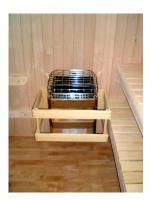
Step 9: Install heater guard around heater making sure that it is evenly spaced around the heater and not touching the heater directly.
